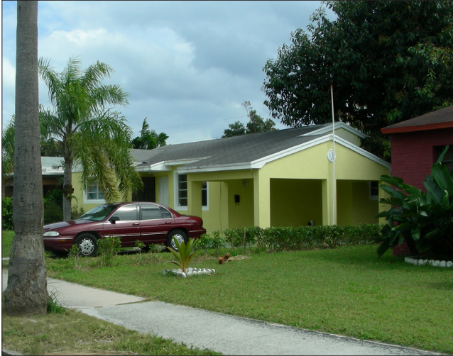
Vehicular access is generally provided via a front driveway and parking is most often provided within the front yard setback or to the side of the primary structure, sometimes in a carport.
