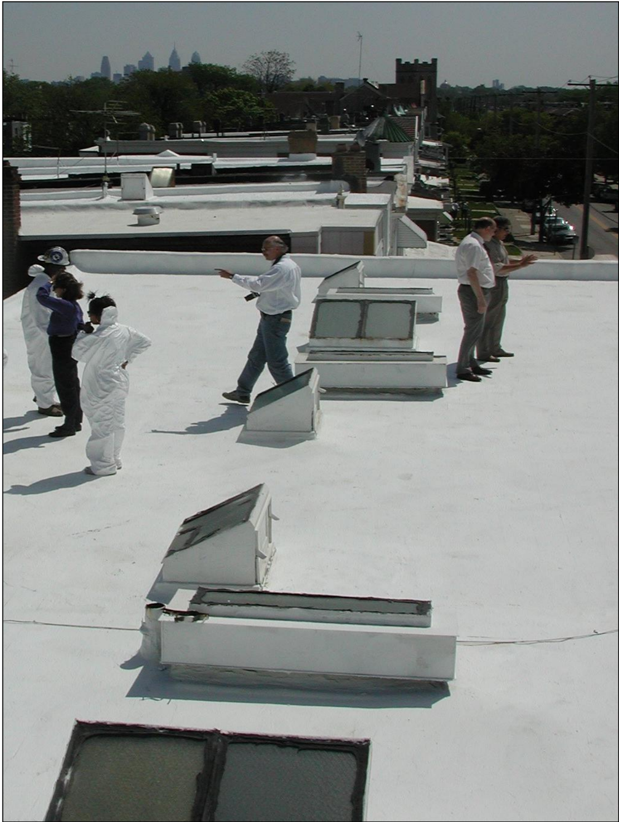
Overview of Several Residential Roofs
