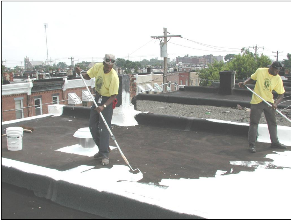
Application of Elastomeric Acrylic Roof Coatings to Residential Roofs
