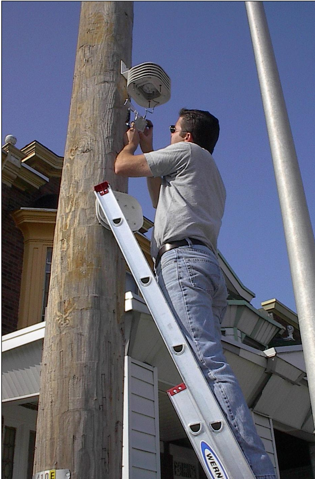
Installing Data Loggers for “Cool Block” Comparison
