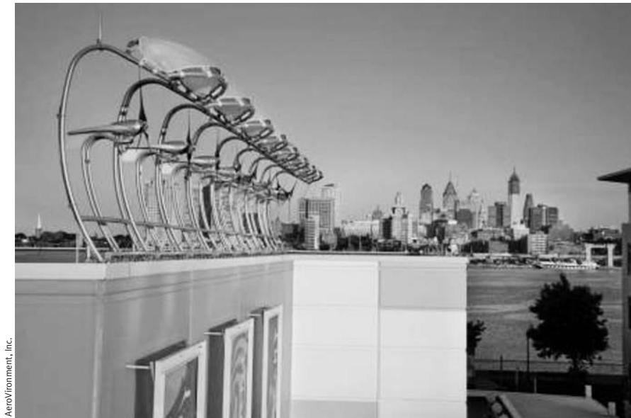
➡ The Adventure Aquarium in Camden, New Jersey, uses a modular, rooftop-mounted turbine system that eliminates the need for stand-alone support towers.
