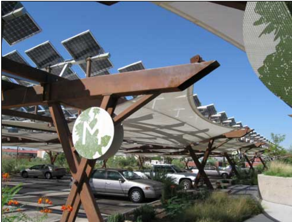
An aesthetically pleasing solar parking lot In addition to generating electric power and shading the cars, this parking lot can charge electric vehicles.
