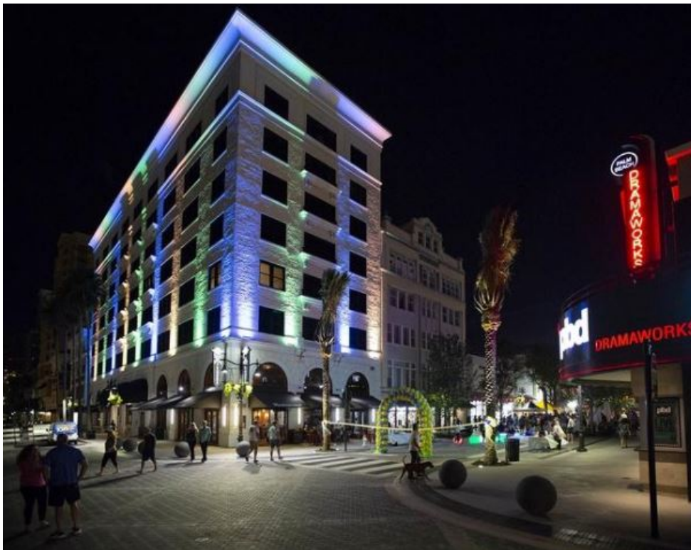
Clematis Streetscape (200 Block)
