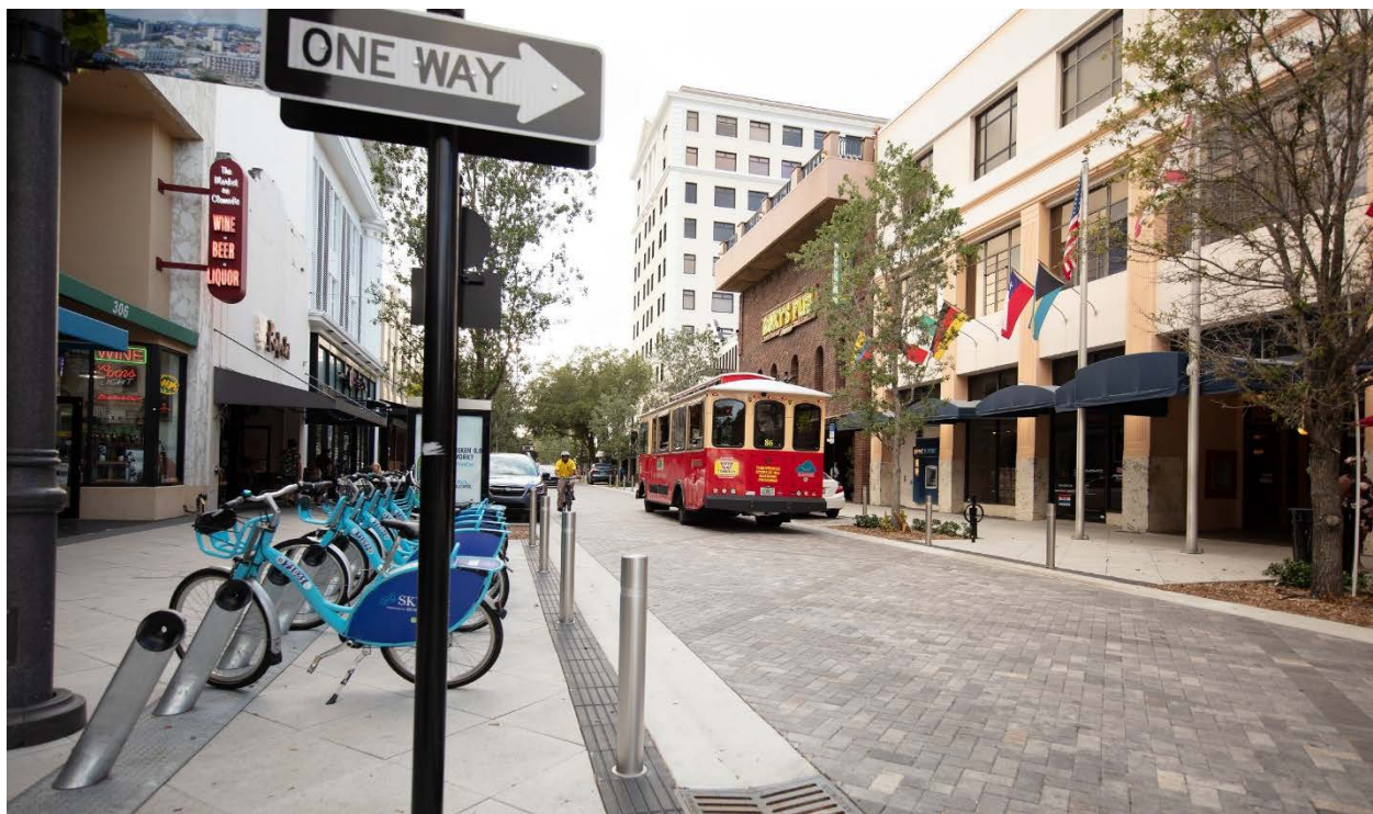
Clematis Streetscape (300 Block)
