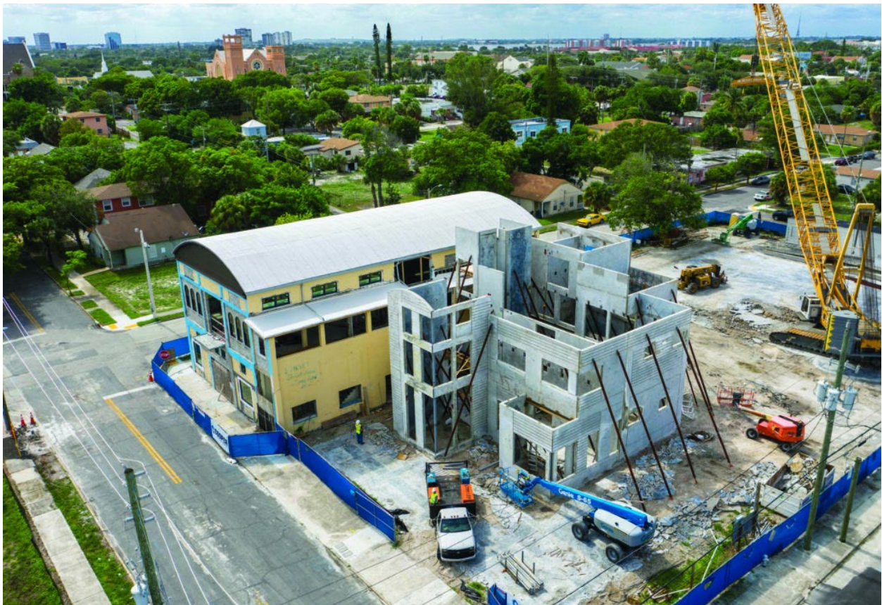
Sunset Lounge (under construction)
