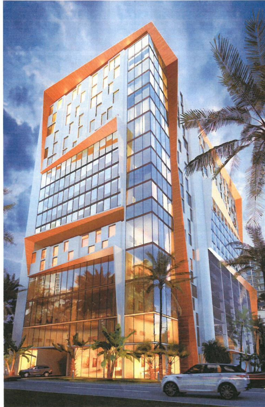
BUILDING 1 VIEW FROM S. QUADRILLE BLVD. 1/17/2015
