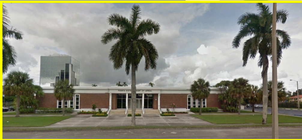
Existing building on PBLakes
