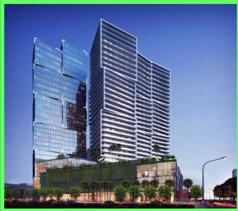
One West Palm Jeff Greene Under construction 206,706
