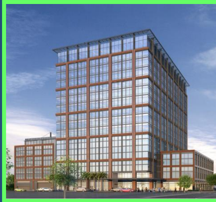
360 Rosemary Related Under construction 258,449 sf
