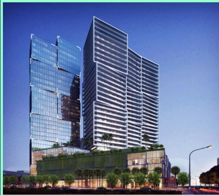
One West Palm Construction underway 200 rooms
