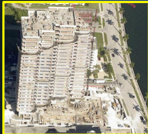
1 LaClara Nearing Completion 1515 S. Flagler
