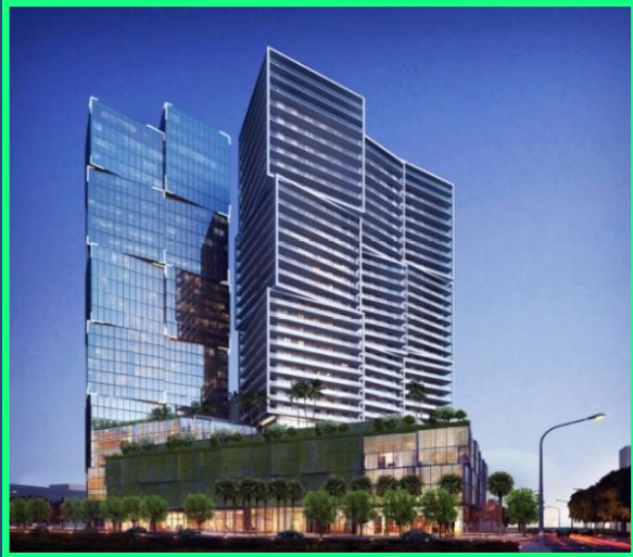
One West Palm In Construction
