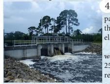
As the water continues down the M-Canal, it passes through Control Structure 4, which can have the gates open or closed depending on the water levels of the lakes.
